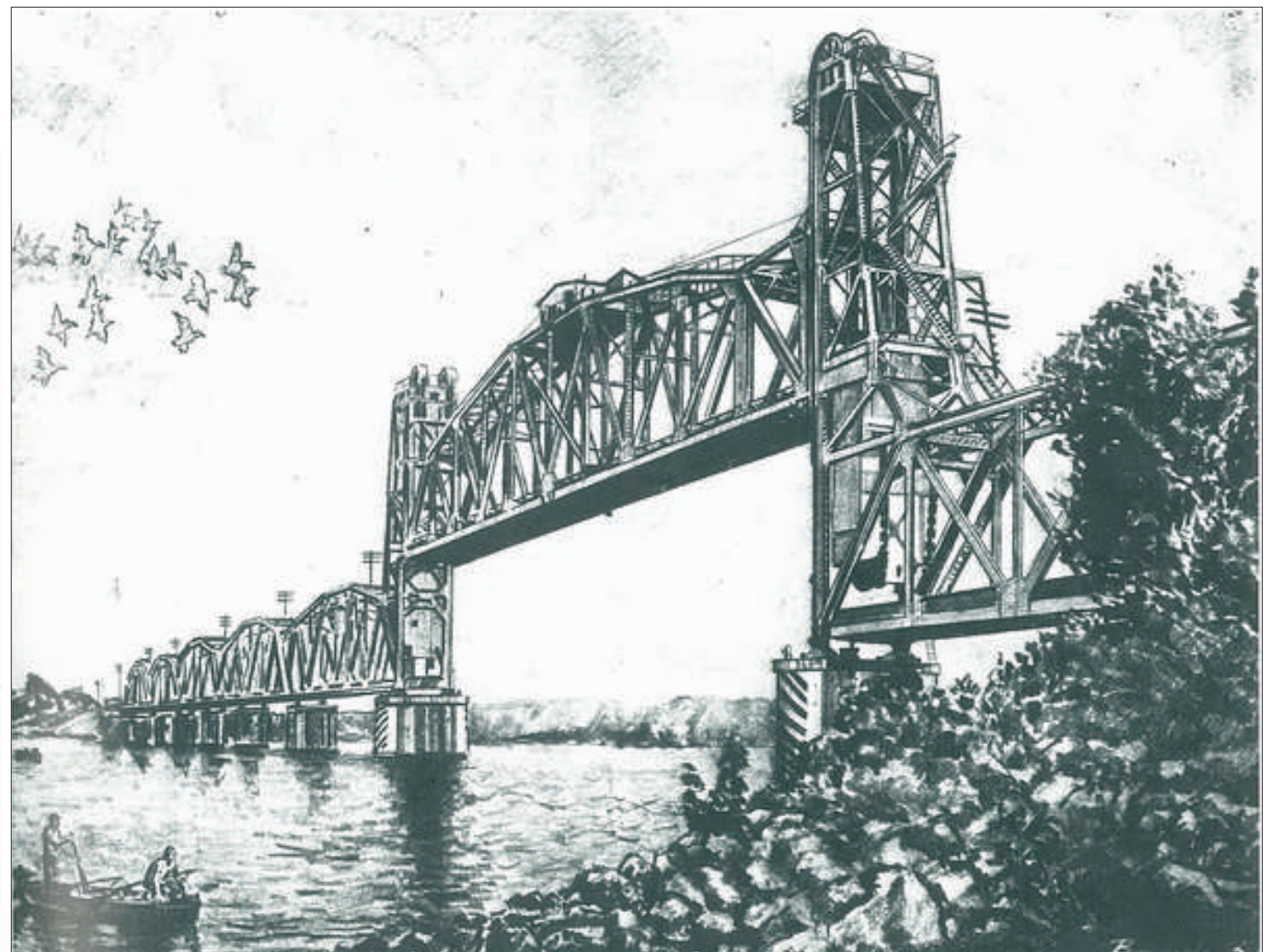
The Danville Bridge
